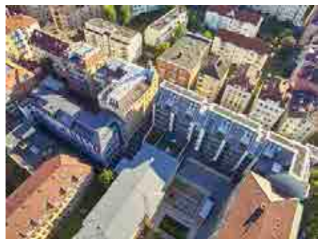
图12 罗特街新建沿街住宅和后院住宅 Fig.12 Apartments along Roetestrasse and in backyard 资料来源:德国CIP公司拍摄。
