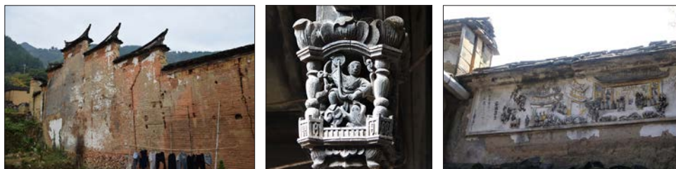
图7 康里村民居建筑的山墙、吊桶与灰塑 Fig.7 Gables, hanging buckets and plaster sculptures of residential buildings in Kangli Village
